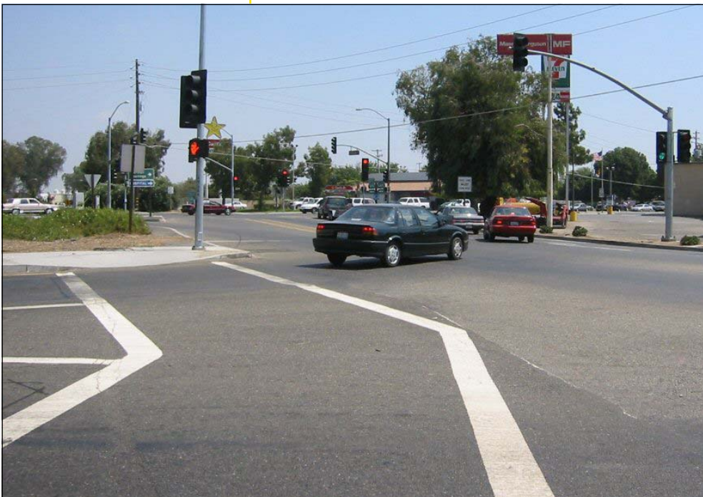
The Madera Avenue project will include widening the intersection at Madera & Olive Avenue.
